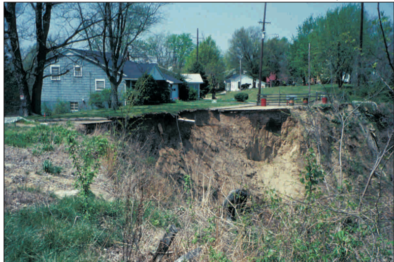
Magnolia Street in Hickman, Ky., was damaged and later collapsed as a result of a landslide.
