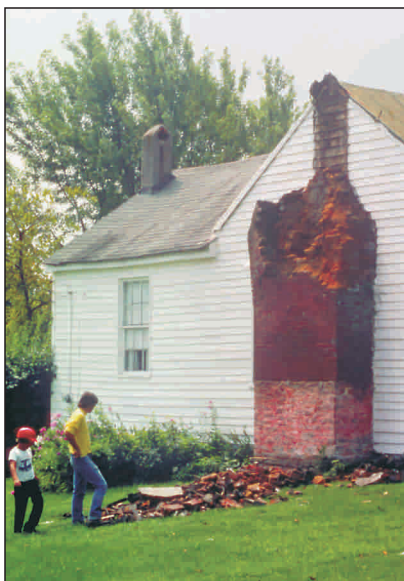
Chimney damage from the 1980 Sharpsburg quake.
