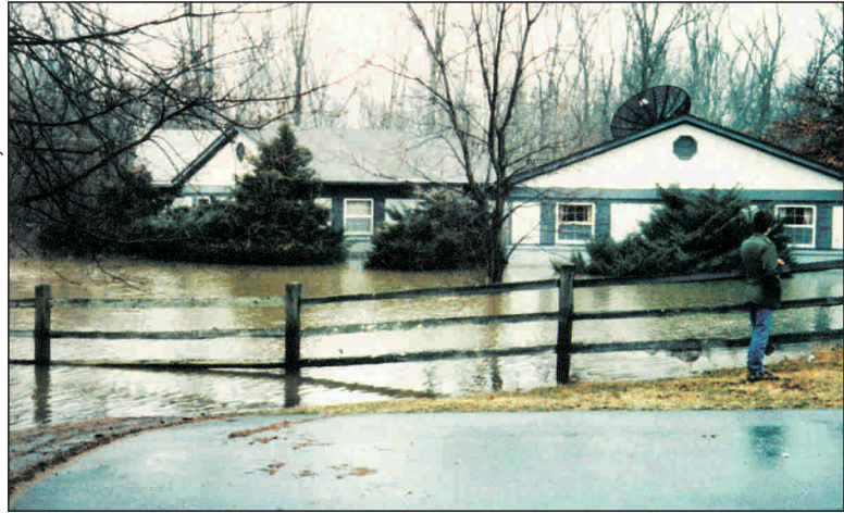
This house in central Kentucky was built in a large sinkhole that has flooded repeatedly since 1989. The sinkhole in which it was built was so large that it was not recognized at ground level as a closed depression. The outlet from the sinkhole cannot accommodate peak runoff from upstream, so during heavy rainfall, it floods. Knowledge of the surrounding area or consulting a topographic map would help a homeowner be alert to such a hazard.
