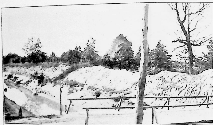
NO. 14. DRAINAGE DITCH.
