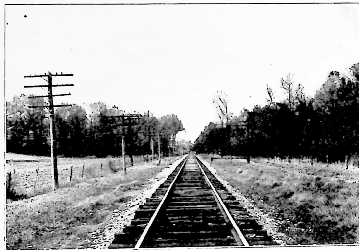
NO. 6. ABANDONED STREAM CHANNEL OCCUPIED BY RAILWAY.
