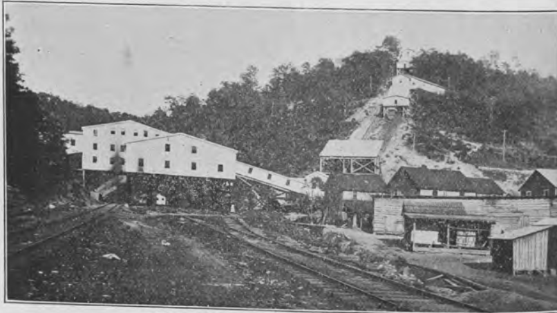
THE HARDY-BURLINGHAM MINING CO. This operation is located in the heart of the Hazard coal field on the North Fork of the Kentucky River at Harburlly, Ky. A double or two track tipple shown the left with mines on either side.
