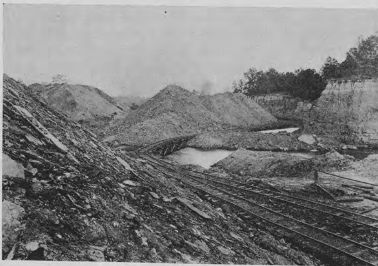
A STRIPPED OUT AREA.
