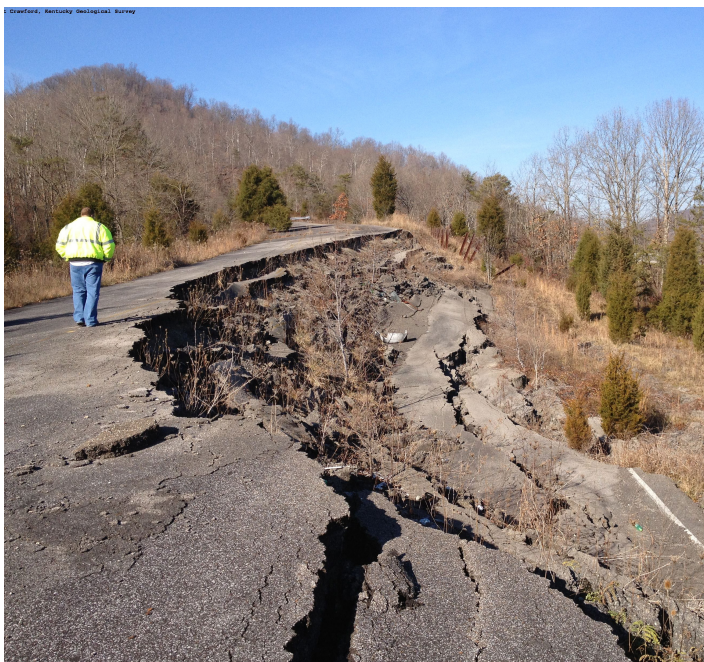
Landslides can be far more than cosmetic—they can block roads, damage utilities, and disrupt entire communities. This 2012 slide in Lewis County highlights the risks of unstable slopes in Kentucky.
