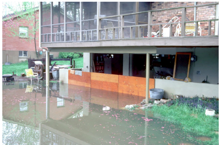
When heavy rain hits a karst landscape, sinkholes and underground channels can’t drain water fast enough. The flooding gets worse when development fills in natural drainage paths. In some cases, the only safe fix is moving houses out of the floodplain. Photograph by Jim Rebmann, Lexington-Fayette Urban County Government.
