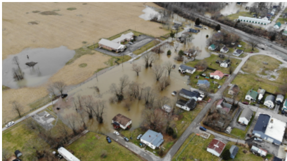
Figure 9. Aerial drone photograph showing flooding impacts in the karst sinkhole valley in Burgin, Kentucky, February 7, 2025 (courtesy of the City of Burgin).
