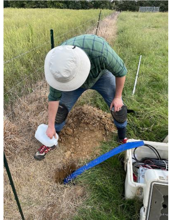
Jon Schmidt uses water to help sand settle around a broadband seismometer installed at the KSSMN station FMKY (Hickman County). Data from this and other temporary installations are helping KGS seismologists to improve KSSMN signal quality.
