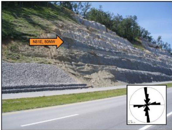
Exposure of jointed Borden Formation along the Bluegrass Parkway in Hardin County. The rose diagram shows joint orientations measured at the exposure, and the orange arrow shows the orientation of one of the joints.
