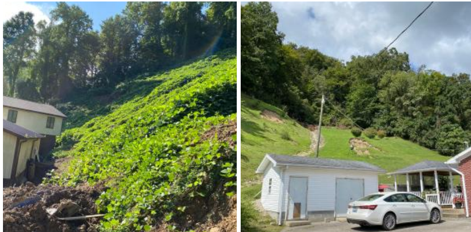
Figures 19 and 20, left to right. Fig. 19: Home damaged by landslides/slumps occurred on the cut slope. There is no or little buffer between the house and slope. Fig 20: Measures preventing landslide damage to home. There is a large space and a concrete wall between the house and cut slope. Also, there is a large drainage to divert the rainwater.
