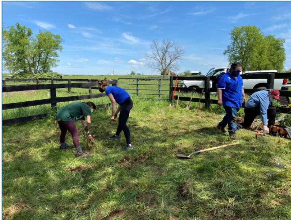
Fieldwork to install permanent electrodes in a sinkhole.
