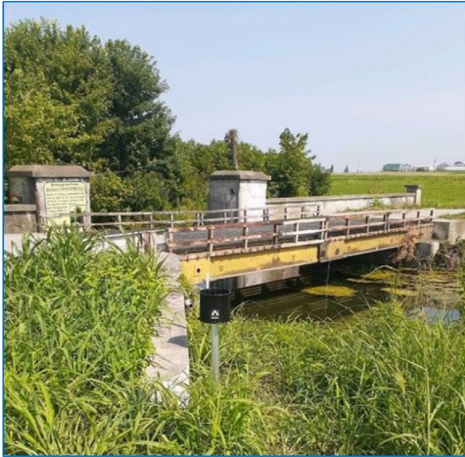
A rain gage and pressure transducer monitoring station installed at Cane Run at Spindletop Research Farm. Photo by Steve Webb .
