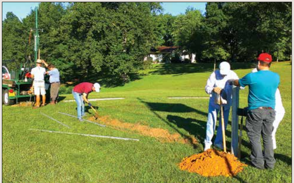
KGS staff, visiting Chinese scholars, and UK students install seismic station EK-22 at the West Liberty Airfield, one of 13 stations in a temporary network to monitor background seismicity as well as induced quakes possibly caused by wastewater injection activities.
