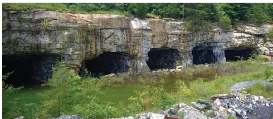
Adits (surface entrances) dug by the Kentucky Rock Asphalt Co. at the Indian Creek Quarry in Edmonson County, about 1927. The company and its operations are among the topics discussed in “Rocks to Roads to Ruin: A Brief History of Western Kentucky’s Rock-Asphalt Industry, 1888–1957,” by Rick Bowersox .
