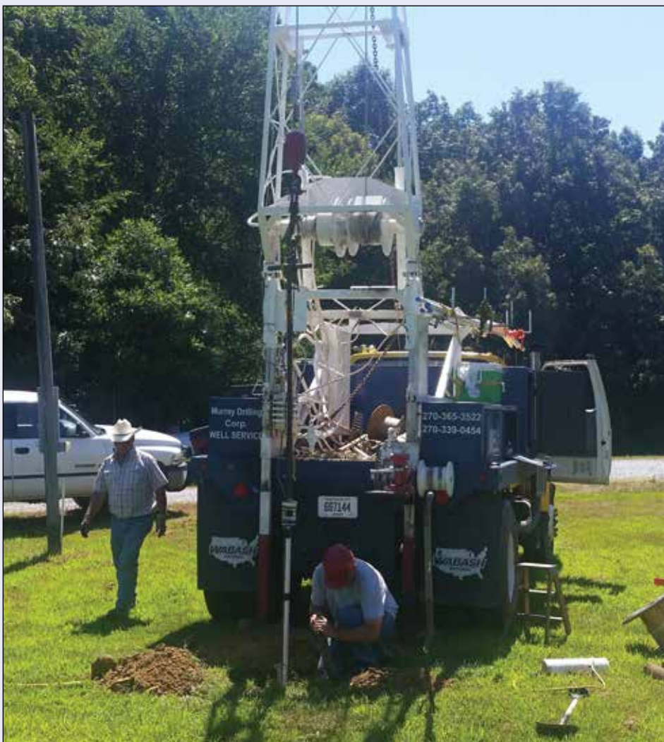
Employees of Murray Well Drilling pull the submersible pump from an unused, 221-foot-deep domestic well in Marshall County. The well is part of the new Kentucky Groundwater Observation Network.
