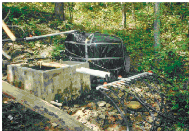
Figure 2. Nonregulated mine-water distribution system. Water is transported into a large cistern equipped with a 12-valve manifold; each individual supply line leads to one or more households. The cistern is covered with black plastic to block sunlight and control algae growth. Overflow at the top of the cistern prevents freezing in winter.
