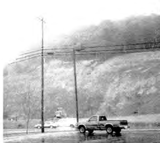
Figure 20. Hillside exposures of highly fractured Breathitt Formation behind motel at stop 8.
