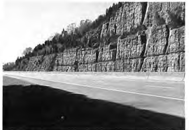
Figure 14. Large fractures and massive bedding in the Camp Nelson Limestone. Note the kink fold and faulted zone in the left part of the picture.
