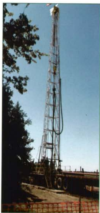
A rig is set up to drill the 1,900-foot-deep hole for the Central U.S. Seismic Observatory.
