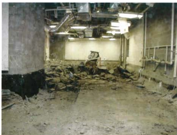
Excavation and repairs were necessary at this Estill County school, where expanding shales damaged the foundation. KGS researchers are studying the problem in this and other buildings in the county.
