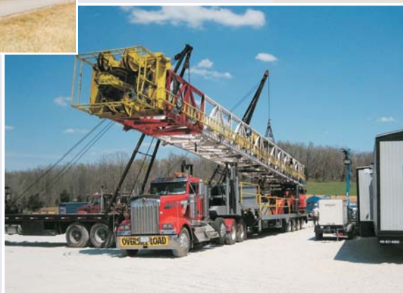
Drill rig arrives
