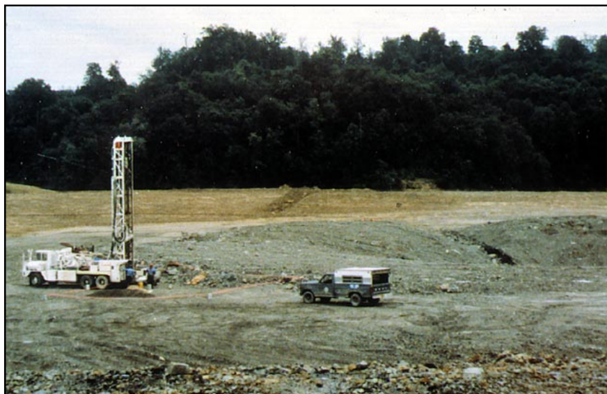
Drilling a monitoring well in eastern Kentucky.
