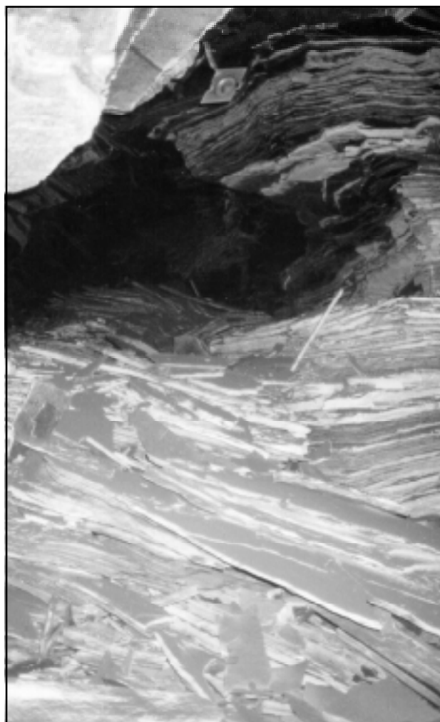
Fall in stackrock roof in an underground mine in eastern Kentucky. Photo by Steve Greb.
