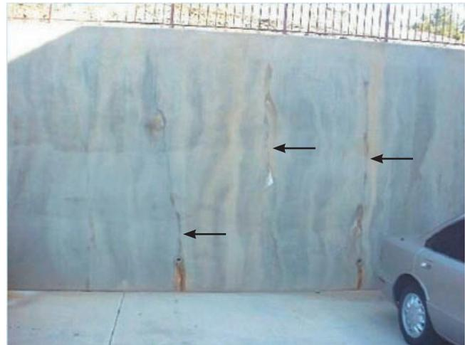
Figure 19. Tension fractures (arrows) along exterior retaining wall and iron-stained drainholes.
