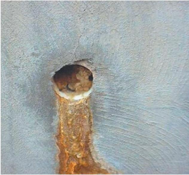
Figure 20. Drain-pipe precipitates (sulfates).
