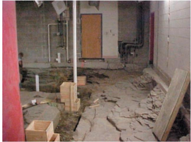
Figure 15. New trench constructed in shale subcrop beneath the middle school. The sulfate mineral copiapite has formed in cleats. Note that load-bearing walls on the right side of the photograph and in the background do not show any signs of failure.
