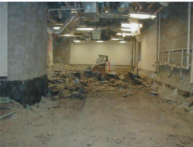
Figure 14. Repair of heaving floors in middle school gymnasium. The original foundation and fill had to be removed and sealed with a resin to prevent further oxidation and heaving of the shale. Photograph by John F. Stickney, Kentucky Rural Water Association.
