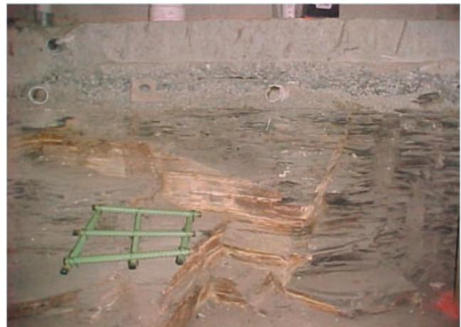
Figure 16. Multidirectional cleat fractures coated with secondary sulfate precipitates such as jarosite, copiapite, and melanterite in the Chattanooga Shale beneath flooring at the middle school. The sewer drain tile was broken by heaving floor slabs, and subsequently was removed. Rebar is being inserted into reinforced concrete columns.
