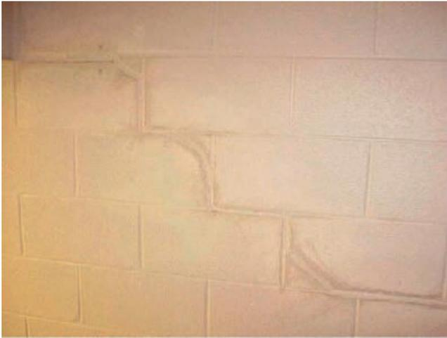
Figure 13. Repaired masonry block cracks.
