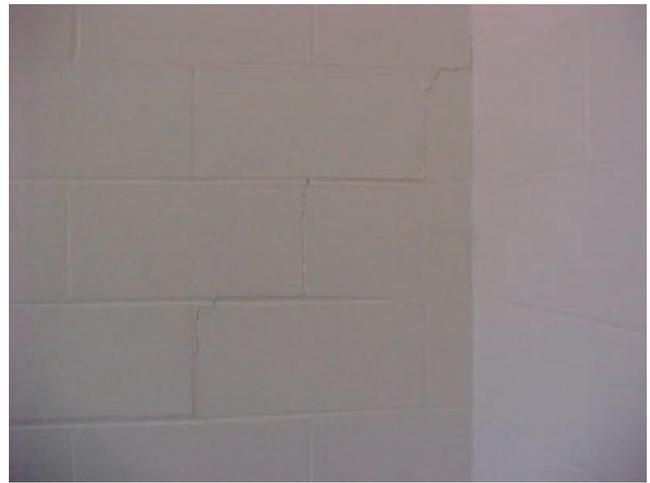
Figure 28. Cracks in concrete blocks at hospital.
