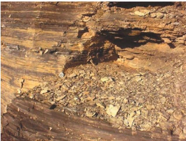
Figure 10. Intersection of pyrite zone with cleat zone in Chattanooga Shale at the middle school. Note extreme weathering of the shale.
