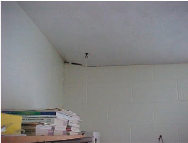
Figure 27. Displacement of ceiling wallboard at hospital along nonload-bearing walls caused by floor heaving.
