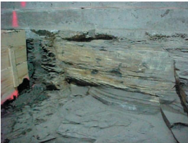
Figure 18. Cleats with sulfate precipitation in shale subcrop beneath the middle school, along with forms for construction of new concrete columns.
