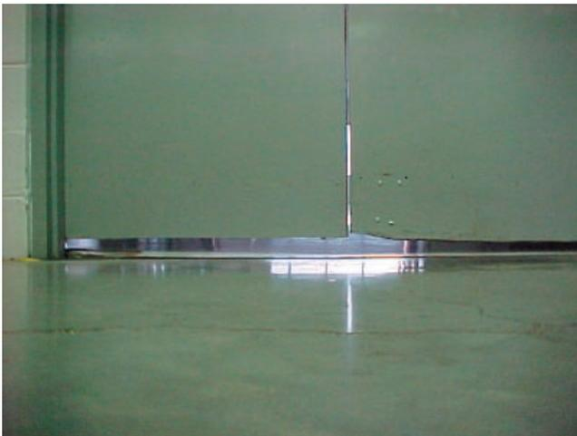
Figure 23. Doors in the Carhartt factory were cut so they could open and close.
