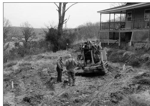
A work crew prepares to drill holes for instruments at the site of the Boyd County landslide that Matt Crawford studied for a year.
