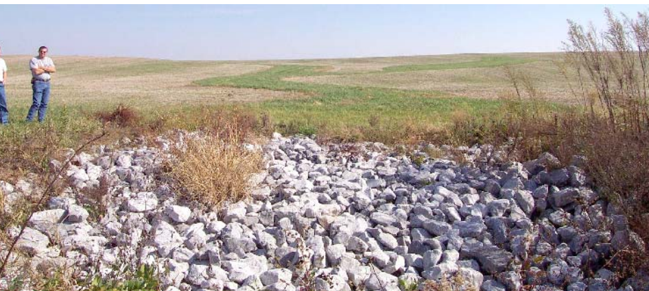
A typical way to control gully erosion, which is very common in Hickman County, is to construct a grassed waterway with a rock chute outlet. Funding for this structure is provided by the CRP CP-21 program through the USDA Conservation Reserve Program. Photo by Glynn Beck, Kentucky Geological Survey.
