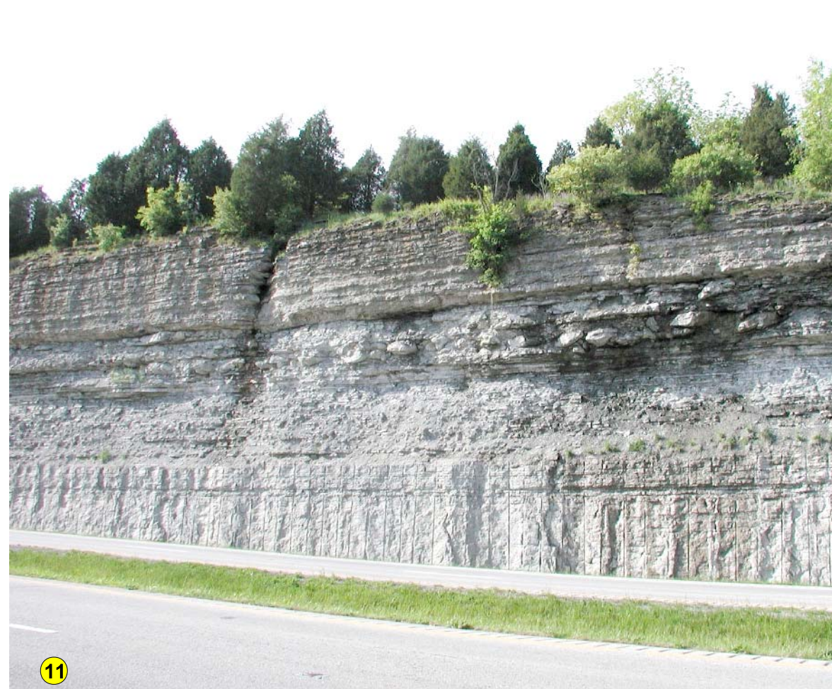
Limestone units 5 and 6 may contain strata mixed with shale, which is more erodible, as seen in this road cut along the Martha Layne Collins Bluegrass Parkway. Photo by Dan Carey, Kentucky Geological Survey.
