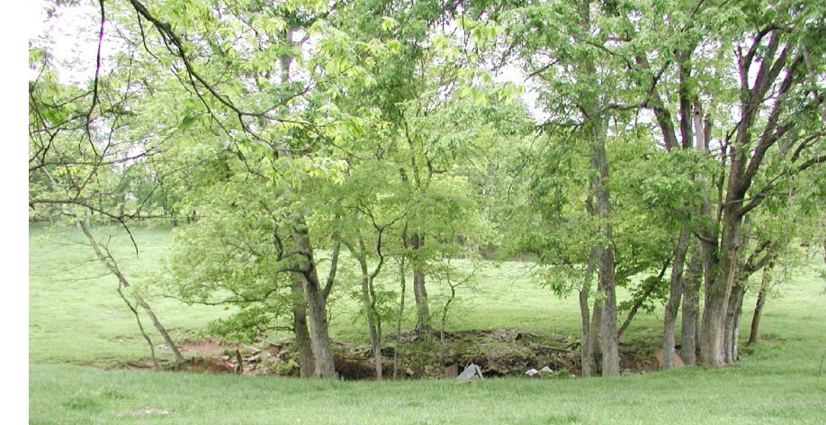
Using sinkholes for waste disposal, even in rural areas, can threaten valuable water resources. Photo by Dan Carey, Kentucky Geological Survey.
