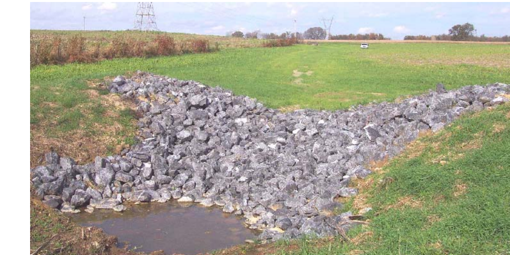
A typical way to control gully erosion, which is very common in Ballard County, is to construct a grassed waterway with a rock chute outlet. Funding for this structure is provided by the Environmental Quality Incentives Program through the USDA Natural Resources Conservation Service. Photo by Glynn Beck, Kentucky Geological Survey.
