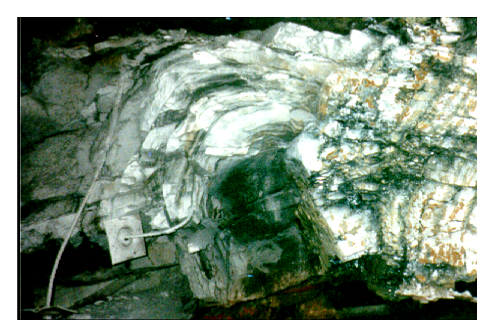
Figure 16. Folding of roof strata toward toe of paleosump.
