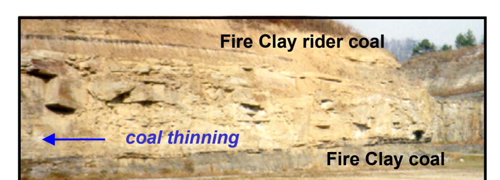
Figure 9. Gradual thinning toward cutout of the Fire Clay coal exposed in a box cut near Hindman.
