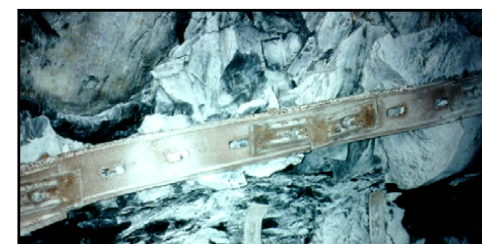
Figure 15. View upward into paleosump roof showing near-vertical beds, slickensides, and jumbled, chaotic bedding.
