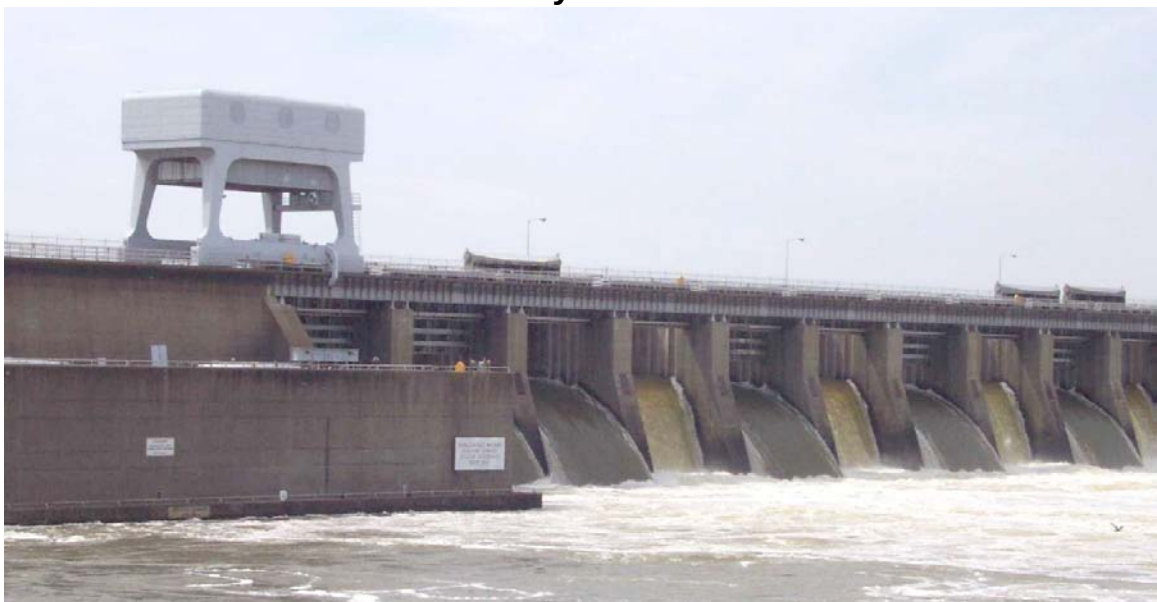
The 60-year-old Kentucky Lake Dam, constructed by the Tennessee Valley Authority on the Tennessee River, is 206 feet high and 8,422 feet long. Kentucky Lake provides flood protection to millions of acres of land along the lower Ohio and Mississippi Rivers. Kentucky Dam also produces hydroelectric power, and has a generating capacity of 184,000 kilowatts. Photo by Glynn Beck, Kentucky Geological Survey.
