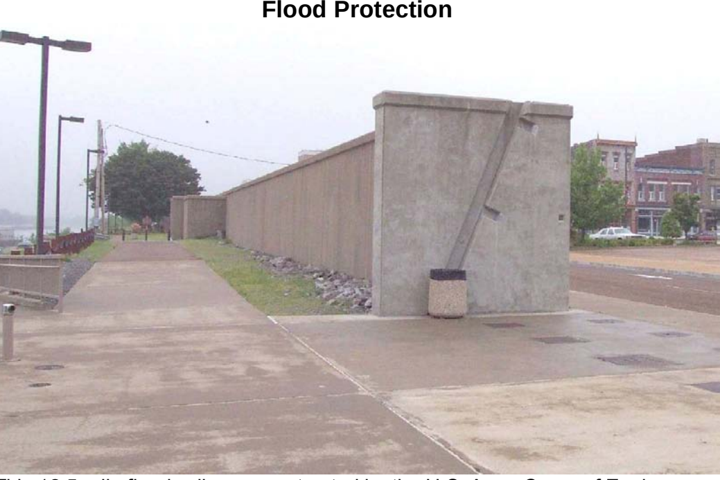
This 12.5-mile floodwall was constructed by the U.S. Army Corps of Engineers after the 1937 flood to prevent future flooding in Paducah. Photo by Glynn Beck, Kentucky Geological Survey.
