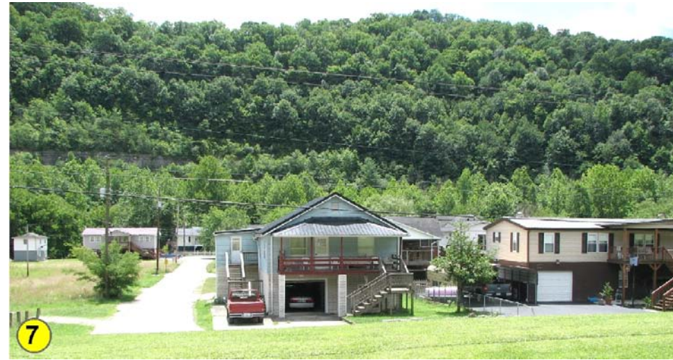
Construction in the floodplain (unit 1) must ensure that living spaces are above flood levels, as shown in these homes along Wolf Creek. Photo by Dan Carey, Kentucky Geological Survey.
