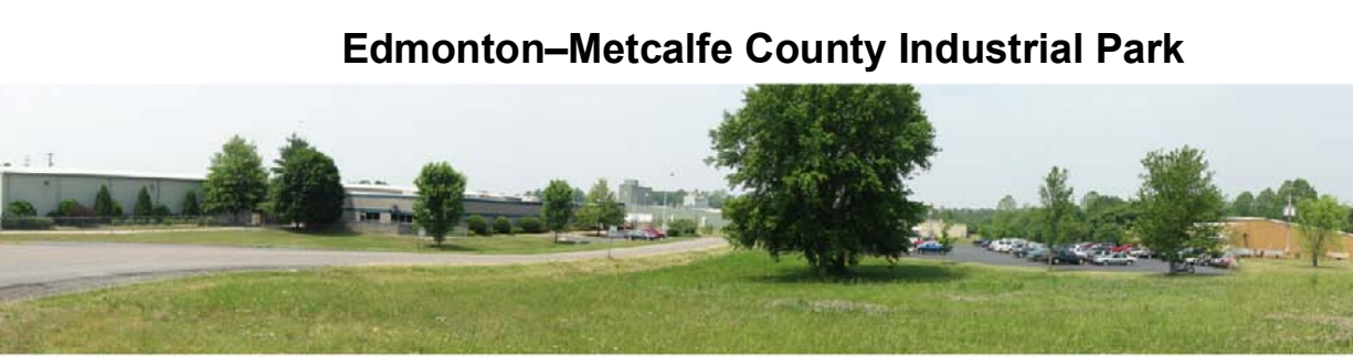
Transportation to and from the 7-acre Edmonton-Metcalfe County Industrial Park is provided by the Louise B. Nunn Parkway (below). Photos by Dan Carey, Kentucky Geological Survey.
