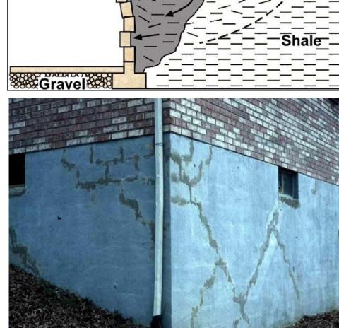
Some shales, and the soils derived from them, swell when exposed to water or air. These swelling shales and soils can have severe impacts on building foundations and other structures (e.g., bridges, dams, roads). Photo by John Kiefer, Kentucky Geological Survey.
