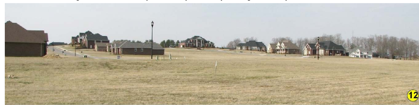
Roaded built on shale (unit 4) requires additional support. Photo by Dan Carey, Kentucky Geological Survey.
