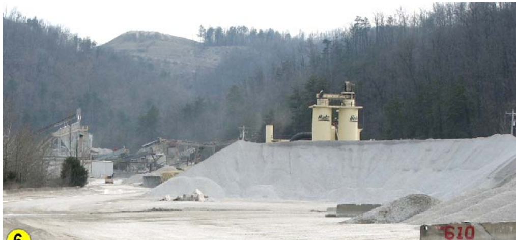
Hinkle Contracting Corporation excavates limestone aggregate from the Stale Formation (unit 4) near Cow Creek Road. Photo by Dan Carey, Kentucky Geological Survey.
