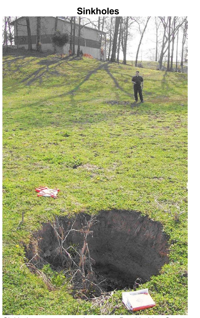
Sinkholes are common in eastern Breckinridge County. They commonly form under or adjacent to houses as small openings, 3 to 4 feet in diameter, as seen above. Without proper management, they can form depressions that are tens of feet in diameter. Photo by Glynn Beck, Kentucky Geological Survey.
