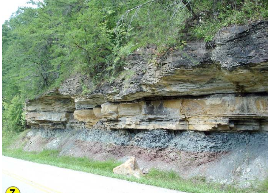
Blue and red shales erode beneath limestone in this roadcut into unit 2 along Ky. 1363. As shale erodes, limestone collapses. Photo by Bethany Overfield, Kentucky Geological Survey.
