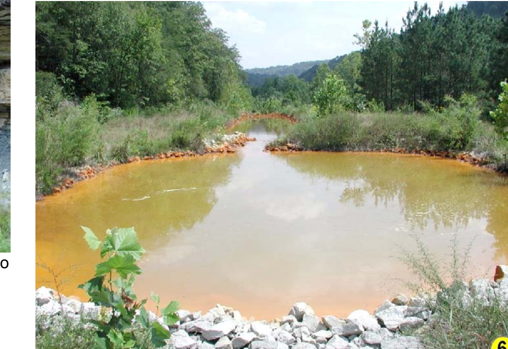
Acid mine drainage from an abandoned underground coal mine is exposed to limestone at this facility, reducing the acidity before it flows downstream. Photo by Randy Paylor, Kentucky Geological Survey.
