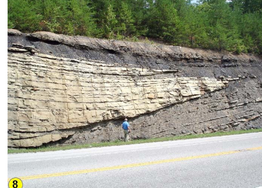
Roadcut along U.S. 27 north of Wiborg shows sandstones over shales in unit 6. Erosion of underlying shale can lead to rock falls. Photo by Bethany Overfield, Kentucky Geological Survey.
