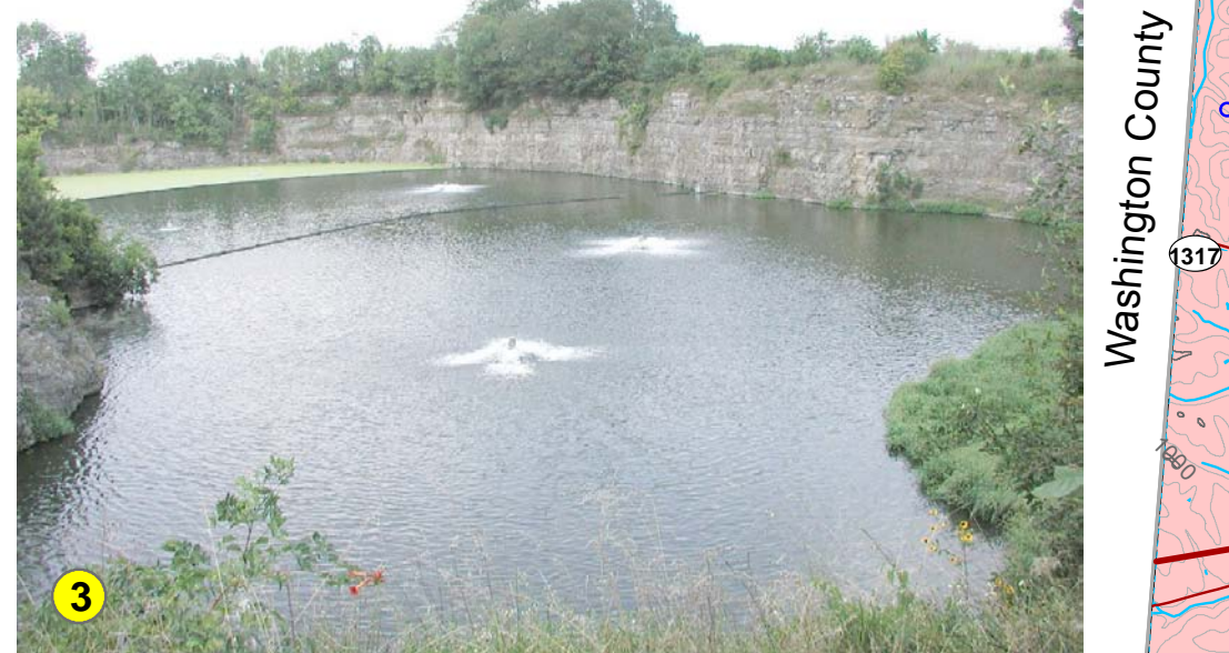
Abandoned limestone quarry off U.S. 68 north of Perrysville has been incorporated into the city's wastewater treatment system. Photo by Dan Carey, Kentucky Geological Survey.
