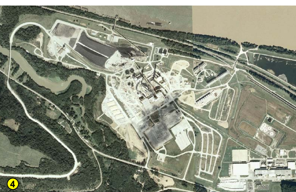
Eastern Kentucky Power produces 1,118 megawatts at the Spurluck coal-fired power station. A second 268-megawatt clean-coal-technology unit will go online in 2008. These units significantly reduce nitrogen oxide emissions, and can burn alternative fuels. Aerial photo (2004) by the U.S. Department of Agriculture, Farm Services Agency, National Agricultural Imagery Program.
