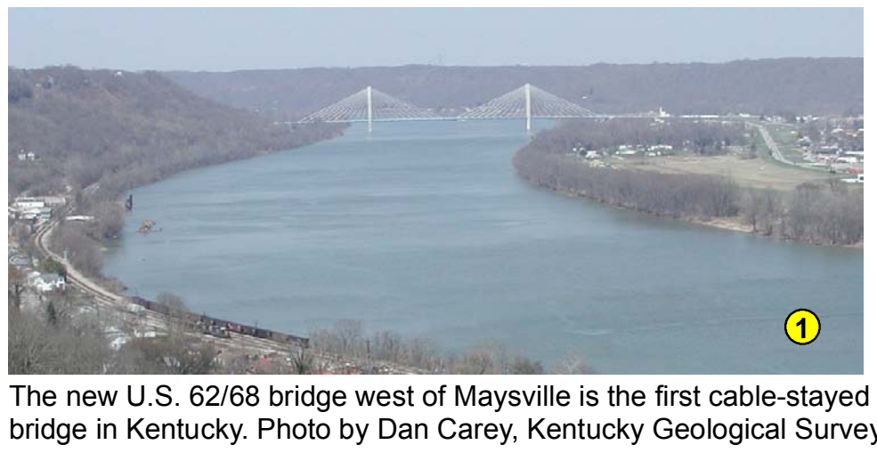
The new U.S. 62/68 bridge west of Maysville is the first cable-stayed bridge in Kentucky. Photo by Dan Carey, Kentucky Geological Survey.
