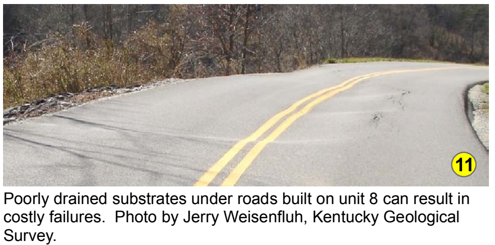
Poorly drained substrates under roads built on unit 8 can result in costly failures. Photo by Jerry Weisenfluh, Kentucky Geological Survey.
