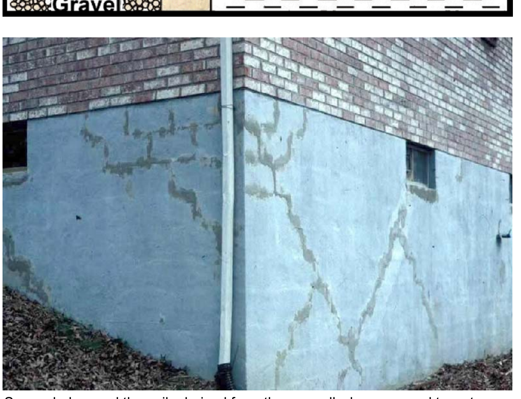
Some shales, and the soils derived from them, swell when exposed to water or air. These swelling shales and soils can have severe impacts on building foundations and other structures (e.g., bridges, dams, roads). Photo by John Kiefer, Kentucky Geological Survey.
