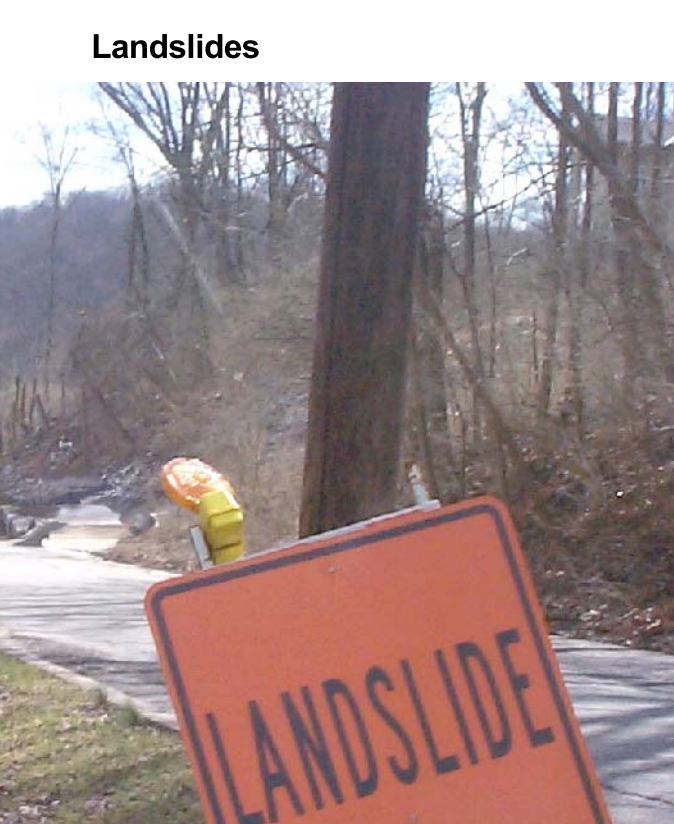
Landslide in the Devou Park area. The toe of the hill was undercut to put in a driveway, and with excess drainage the slope failed. Note the angle of the trees. Photo by Richard Smath, Kentucky Geological Survey.
