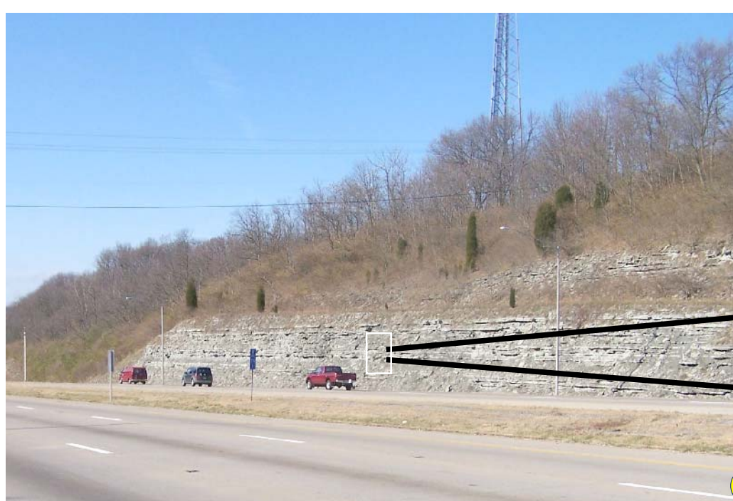
Limestone and shale (unit 3), the 500-million-year-old (Ordovician-age) Fairview Formation, is common as bedrock in Kenton County, and can cause problems for builders because the shales in the unit can swell when exposed to water. Photo by Richard Smath, Kentucky Geological Survey.
