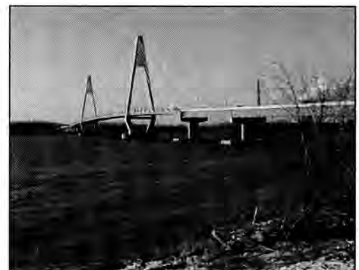
Figure 29. The U.S. 231 Natcher Bridge crosses the Ohio River near Rockport, Ind. The bridge opened to traffic in August 2002.
