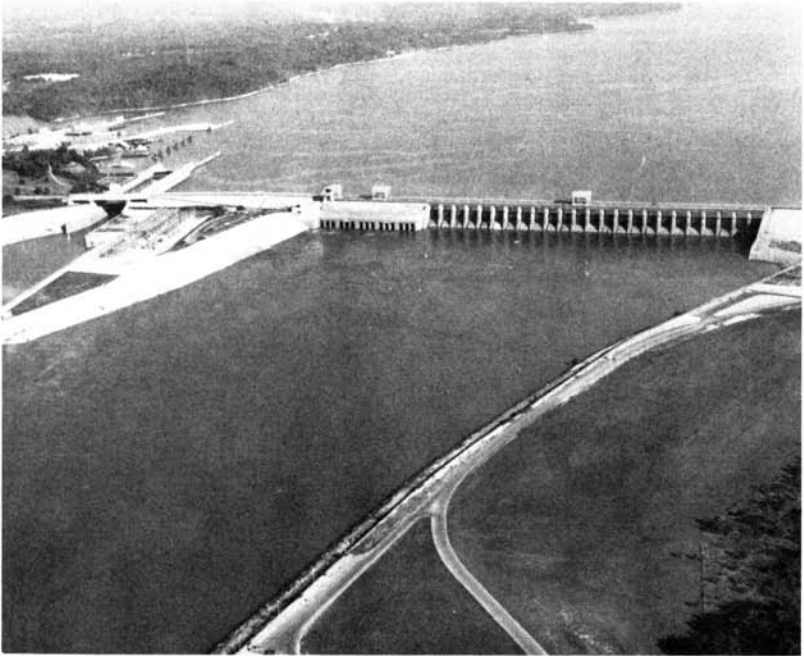
Figure 54. Kentucky Dam, on the Tennessee River in western Kentucky, impounds waters to form Kentucky Lake, the largest in the Tennessee Valley Authority system. The dam and lake are used for flood control, navigation, power generation, and recreation. Kentucky Office of Tourism Development photograph.
