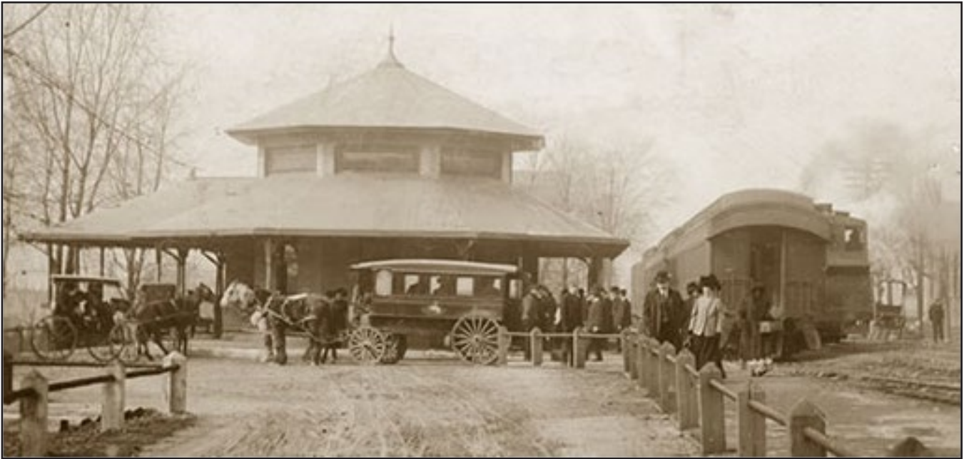
Figure 26. The Madison, Ind., Railroad Station. It was built in 1850 at a cost of $4,094.32. From National Park Service (no date).
