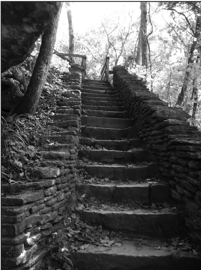
Figure 23. CCC project stairs and wall trail, Big Clifty Falls.
