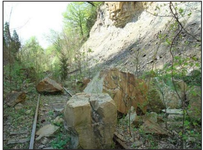
Figure 29. Fallen rocks on the right-of-way, April 2013. The Indiana Department of Transportation was to take bids on restoring the damage and make it safe as a walking trail in October 2013. Failing that, a rails-to-trails recreation trail may be its fate. From Madison Courier (2013); used with permission.
