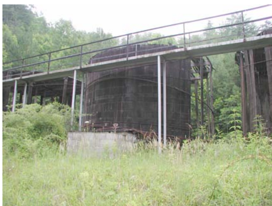
Figure 14. Redwood water filtration and conditioning tanks.
