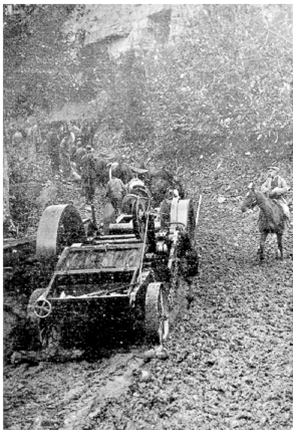
Figure 3. Snagged on the road. Jillson (1919, p. 8) aptly titled this picture to illustrate the difficulties of hauling a rig onto location. This was taken on the road from Torrent in 1918.
