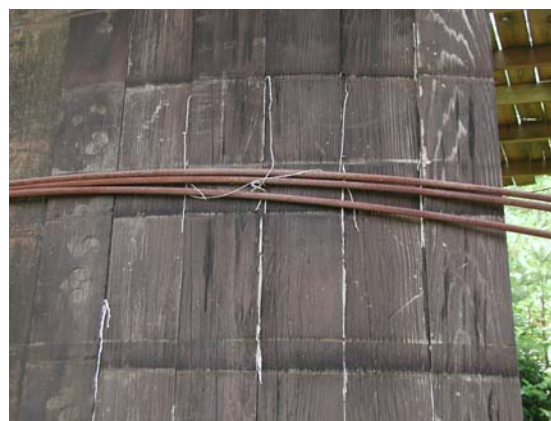
Figure 15. Detail of tank showing string packing between planks.
