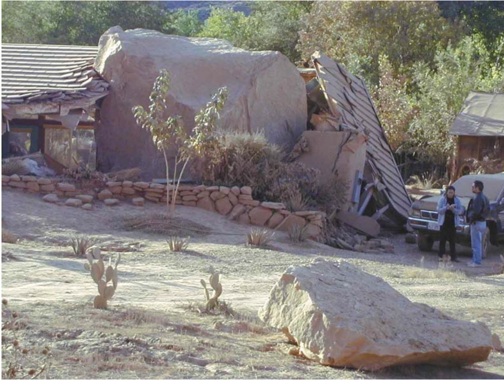
A large boulder that has crushed a building in Zion National Park. (National Park Service photo.)
