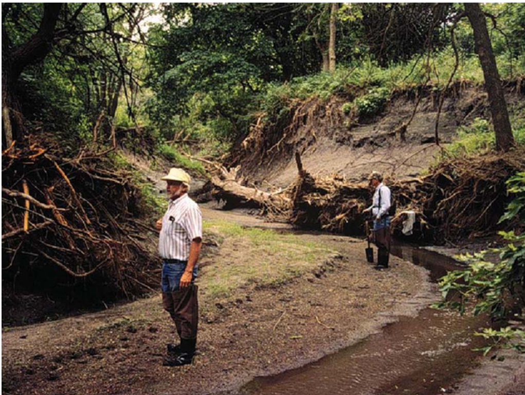
An unstable stream in eastern Nebraska. It has downcut and is widening because of changes in runoff and sediment loads after land use changed from prairie to row crops in the late 1800s.
