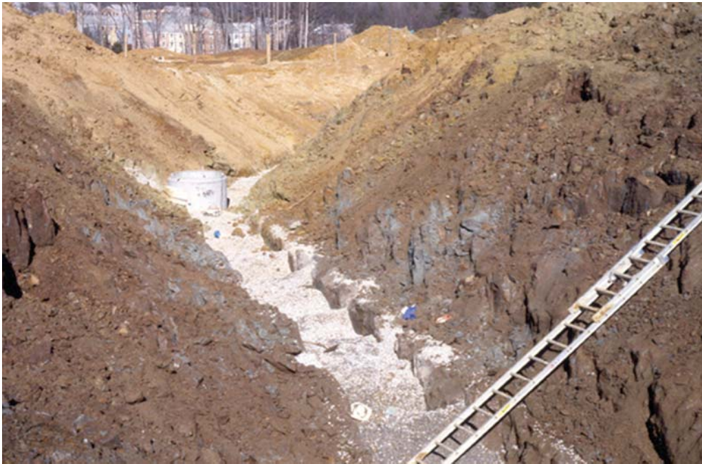
An adequately sloped trench.
