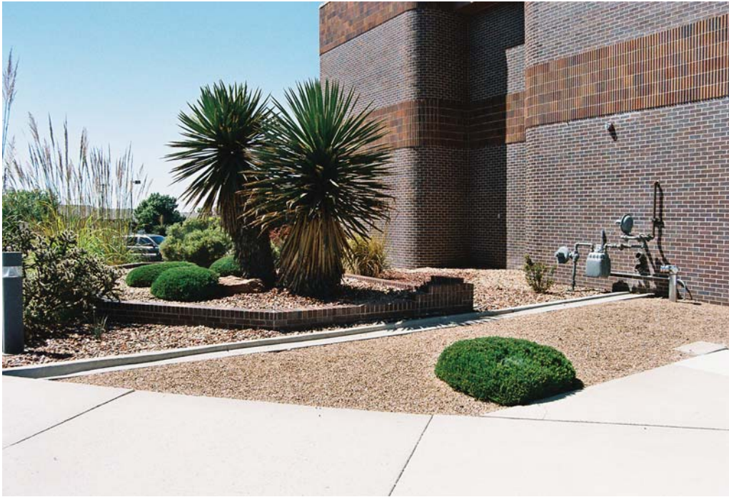
Low water-use landscaping and drainage away from buildings help to prevent soil collapse. (NRCS photo.)
