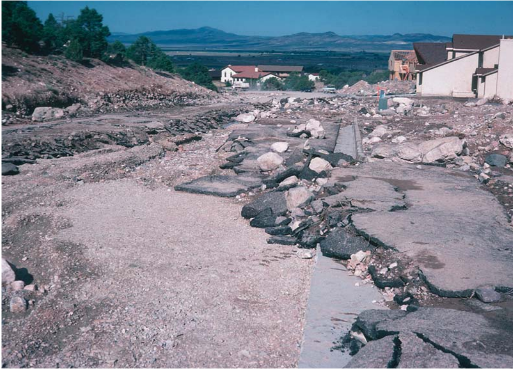
Rocks and debris litter a roadway after a flash flood in Weber City, Utah. (NRCS photo.)
