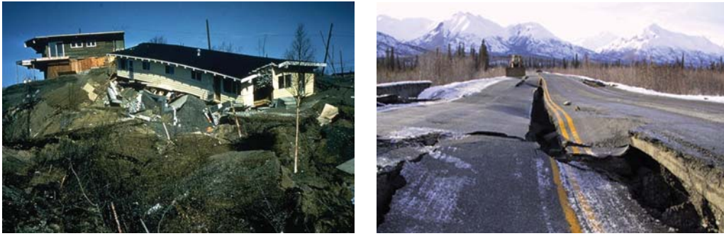
Damage caused by soil liquefaction during a major earthquake. (NRCS photos.)
