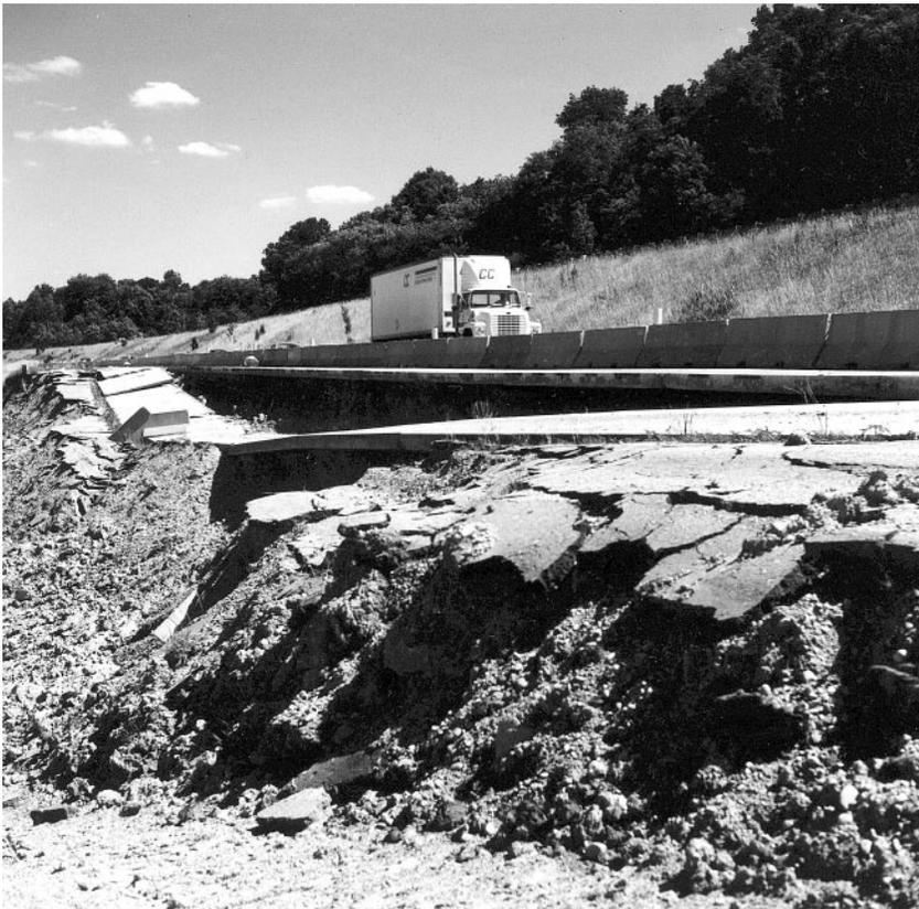
Figure 78. Embankment collapse on Interstate 74 in western Hamilton County, Ohio, undermined by a rotational slide. Highways parallel to hillslopes in the Greater Cincinnati area need special stepped benching or concrete piers in bedrock to minimize such failures (see Figures 79-80).
