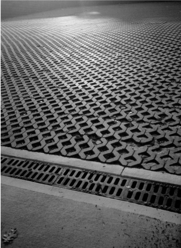
Figure 73. This permeable parking lot still keeps you out of the mud. The open pattern of concrete blocks permits infiltration. These work best where placed above permeable beds.
