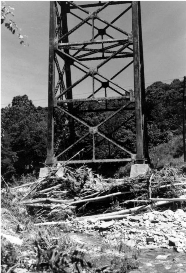
Figure 71. Debris piled against the pier of a trestle of the CSX Railroad over Banklick Creek in Kenton County, Ky., after the flash flood of July 1996. Such floods become both more frequent and intense as impermeable roofs, roads, and parking lots replace fields and woods.
