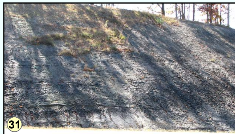
Mile 174.4: Middle part of Breathitt Group (Pbm). Shale, largely carbonaceous, dark gray to black, with ironstone concretions.
