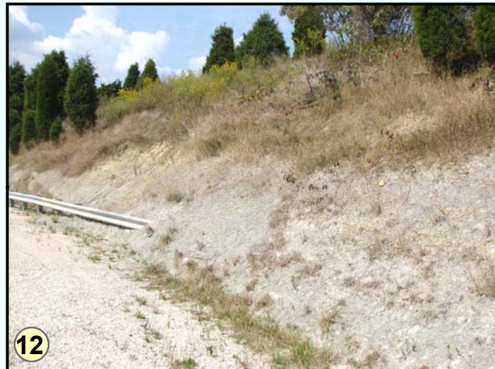
12 Mile 126.2: Green and red Silurian Alger Shale (Sa) is unstable on slopes unless protected by vegetation.
