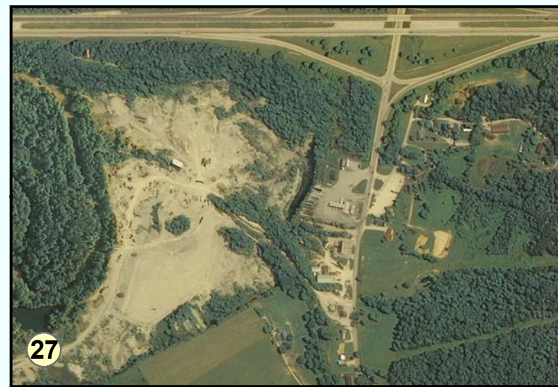
Mile 161.5: Limestone of the Slade Formation (Msla) is quarried for use as crushed stone for road construction and concrete aggregate. Photo from the U.S. Department of Agriculture–Farm Services Administration, National Imagery Program (2004).
