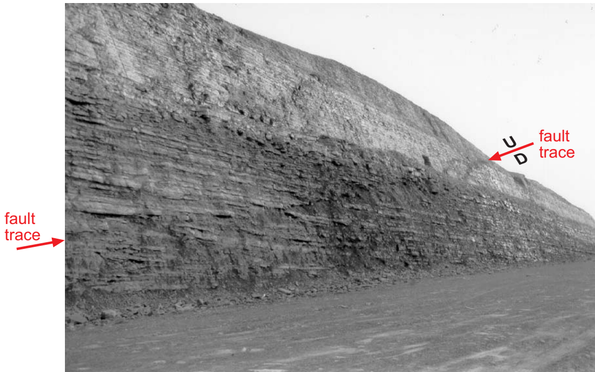
Figure 16. Low-angle fault in the Fairview Formation at mile 2.2 of U.S. 62, Mason County. View is to the south; east wall of roadcut is shown. See Potter and others (2001) for more details.
