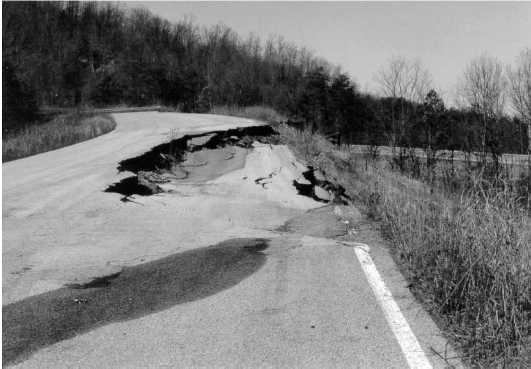
Figure 21. Landslide damage to abandoned Ky. 10, just east of Herron Hill at mile 22.1 of Ky. 9/10, Lewis County. The road was constructed on fill material and colluvium derived from the Crab Orchard Formation. When saturated with water, the fill and colluvium lose strength and slide downslope toward the AA Highway in the background.
