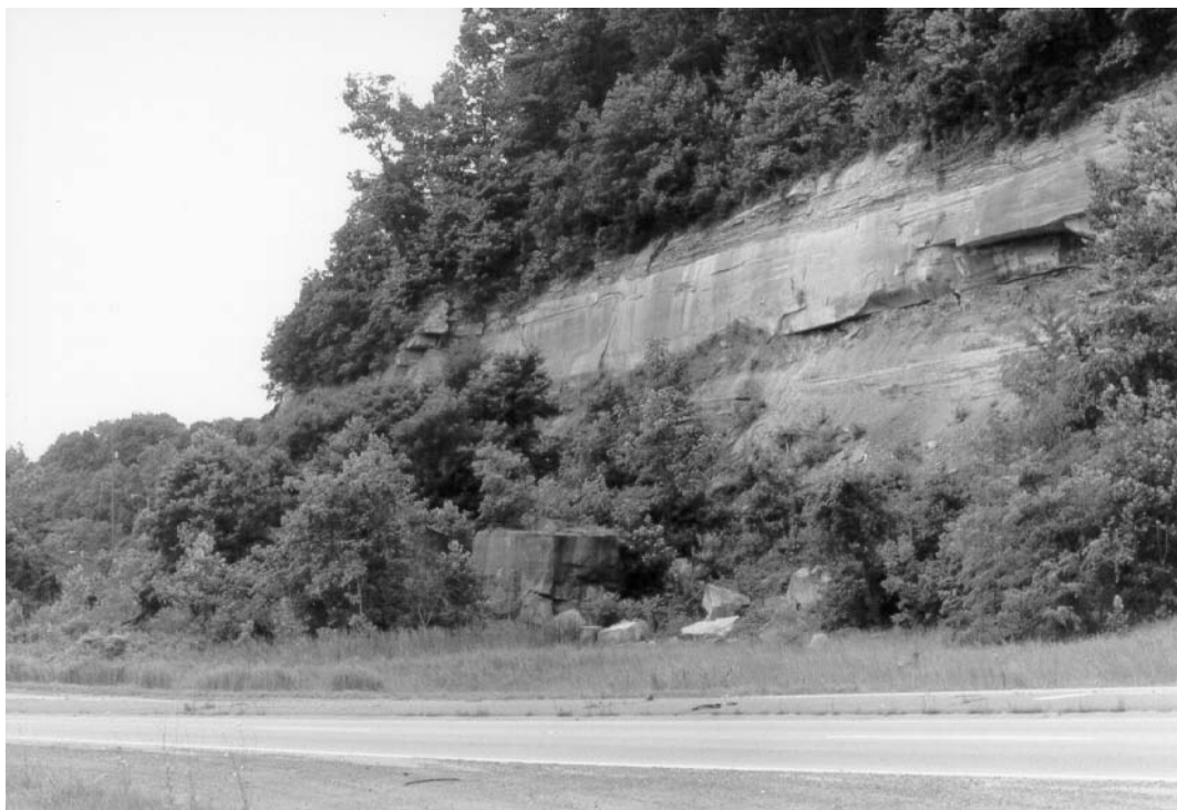
Figure 33. Rockfall of large sandstone block from thick sandstone beds exposed near top of roadcut. Rockfalls occur rapidly and without warning, leading to property damage and loss of life. Overhanging rocks should be removed, where possible, and areas below avoided. Mile 0.6 of U.S. 23, Greenup County.
