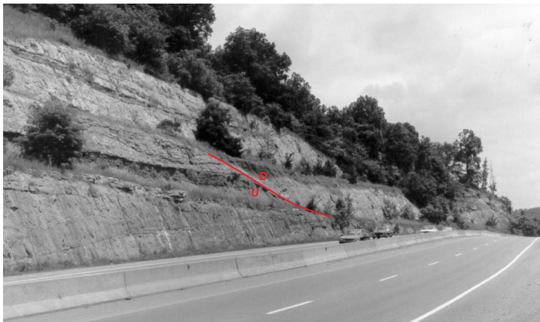
Figure 34. Sandstones, shales, clays, and thin coals of the Breathitt Formation, between miles 19.9 and 19.6 of U.S. 23, Boyd County. The Princess No. 7 coal bed is poorly exposed in this roadcut. Fault present in the middle of outcrop has displaced the prominent sandstone bed downward from its original position.
