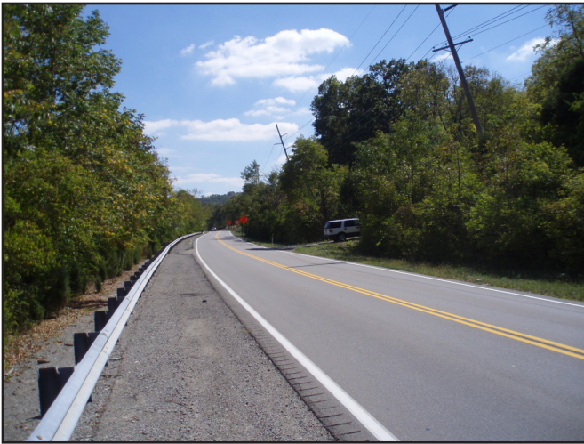
Figure 13. Recently repaired I-beam piers and leaning telephone poles along Ky. 8 are evidence of landslide activity. Ky. 8 is in constant need of repair because of landslide damage.
