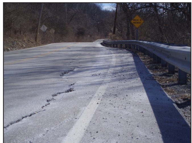
Figure 12. Evidence of landslide activity: The road is benched into the middle of the slope and the landslide stretches above and below the road. There is significant offset in the pavement.
