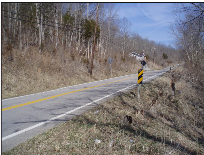
Figure 11. An old I-beam pier retaining wall in the grass suggests previous slope failure, and a leaning telephone pole suggests the slope is actively creeping.
