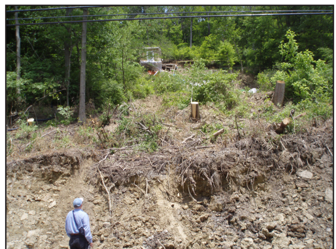
Figure 4. Landslide along Ky. 3187. Thick colluvium is shown at the bottom of the photo and a threatened home toward the top.
