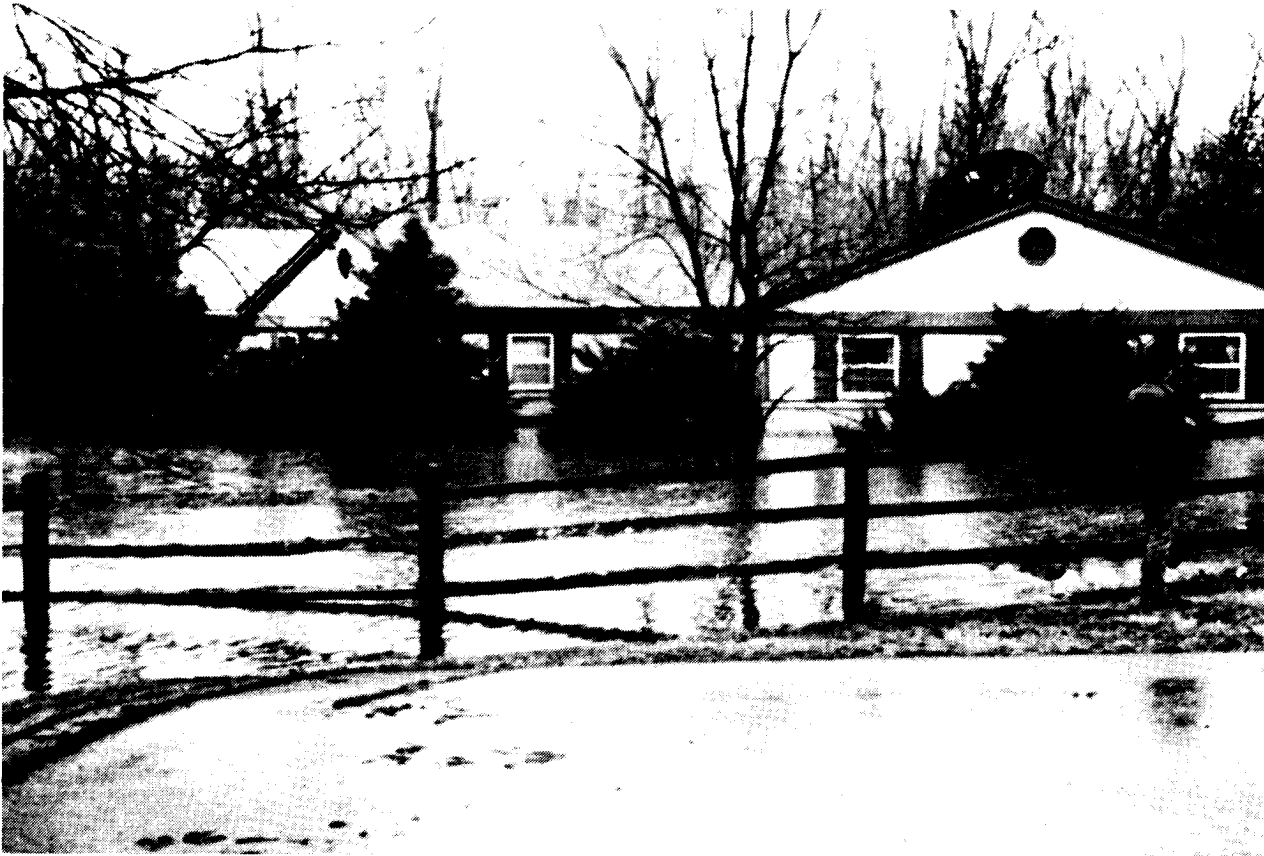
Figure 1. Home damaged during the February 1989 storm. The building is a split level, and 2 to 3 feet of water is in the upper level.
