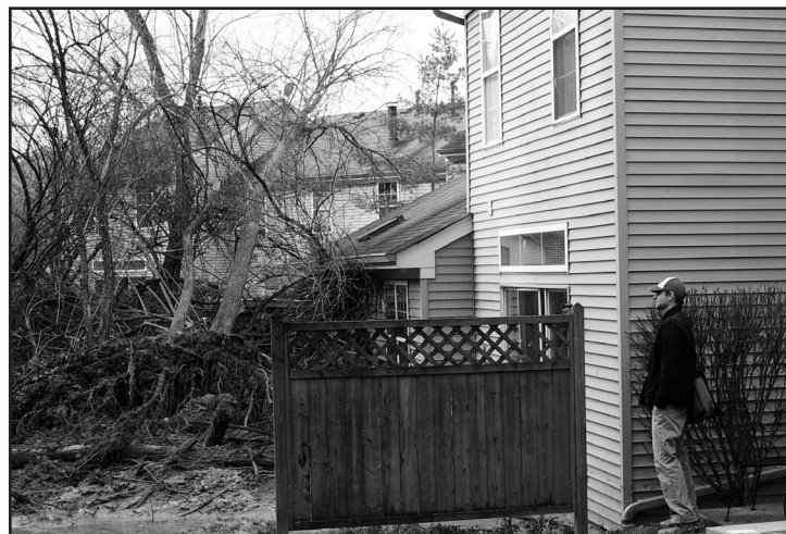
Matt Crawford surveys damages to several condominiums in Bellevue, Ky. The hillside behind the homes suddenly slid after several days of heavy rain in early December.
