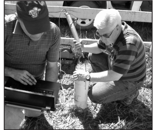
Steve Webb (left) and Section Head Chuck Taylor (right) check the operation of telemetry equipment they installed in a groundwater observation well at the Kentucky Horse Park. It was the first of 14 wells planned for the new groundwater network.
