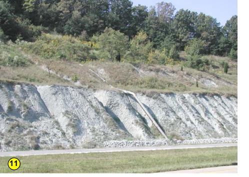
Drainpipes and limestone riprap are used along the shale slopes of the Muldraugh Escarpment to help prevent water infiltration and subsequent slope instability onto the Gene Snyder Expressway. Photograph by Bart Davidson, Kentucky Geological Survey.
