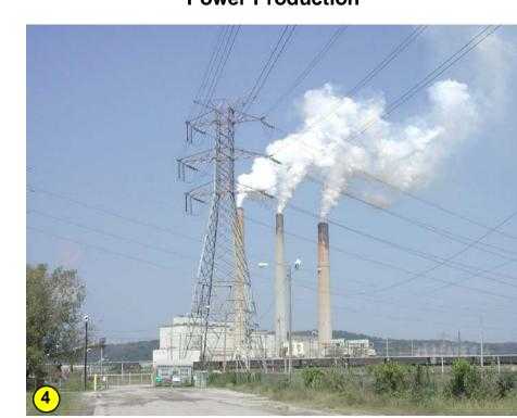
Large cities such as Louisville require great amounts of electricity. Louisville Gas and Electric's Mill Creek Power Station on the Ohio River is a 1600 megawatt coal-fired plant. The flue-gas desulfurization unit at the plant produces half a million tons of gypsum annually as a byproduct that is shipped by barge to a wallboard plant. Photograph by Bart Davidson, Kentucky Geological Survey.
