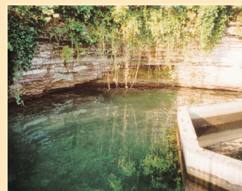
Impounded spring used for a public water supply.
