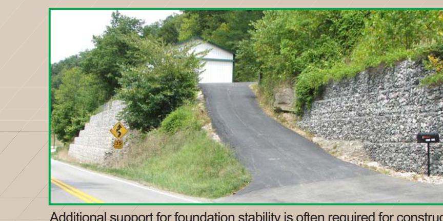
Additional support for foundation stability is often required for construction on slopes (Johnson County). Photo by Dan Carey, Kentucky Geological Survey.
