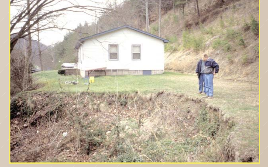
This landslide in Johnson County was caused by a septic drain field. Photo by Paul Howell, U.S. Department of Agriculture, Natural Resources Conservation Service.
