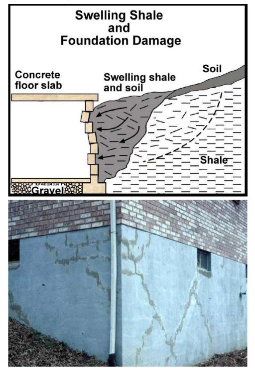
Some shales and the soils derived from them swell when exposed to water or air. These swelling shales and soils can have severe impacts on building foundations and other structures (e.g., bridges, dams, roads). Photo by John Kiefer, Kentucky Geological Survey.
