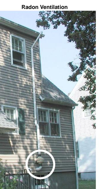
Ventilation system removes radon from the basement area of this home. Photo by Dan
