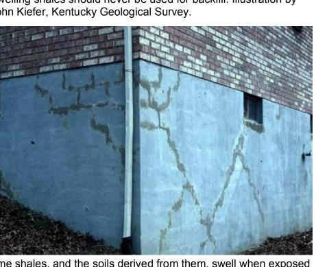
Some shales, and the soils derived from them, swell when exposed to water or air. These swelling shales and soils can have severe impacts on building foundations and other structures (e.g., bridges, dams, roads). Photograph by John Kiefer, Kentucky Geological
